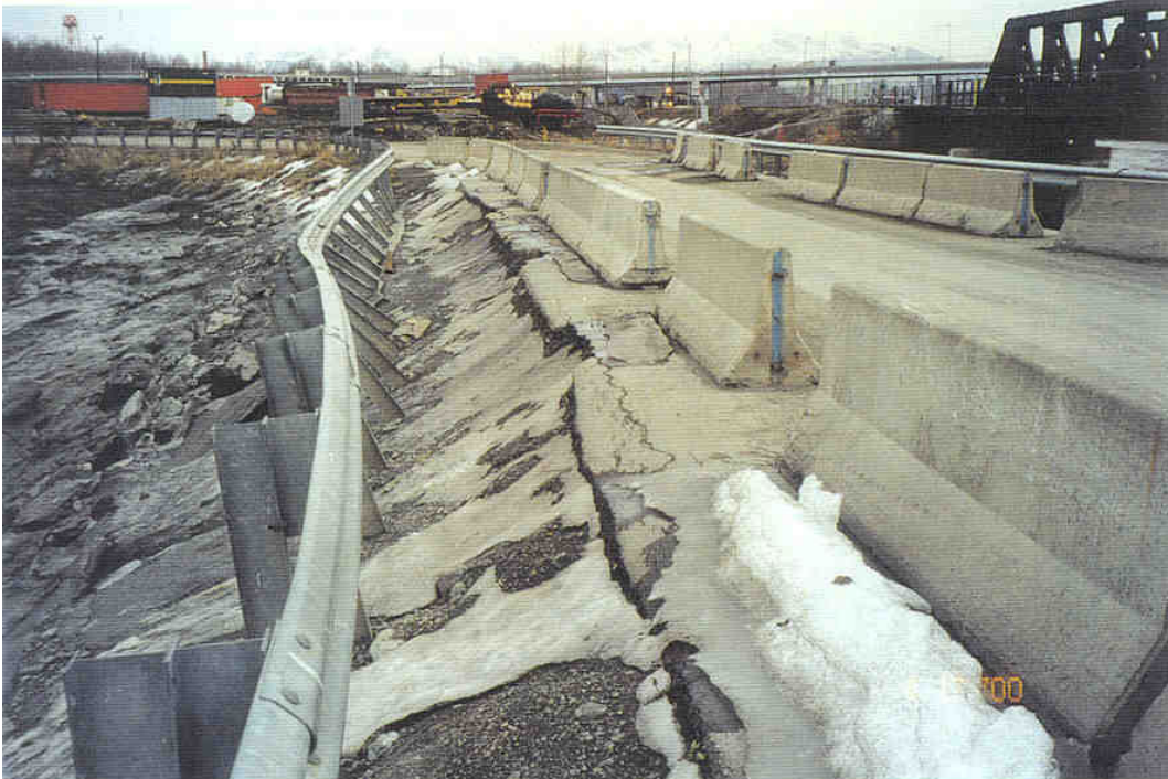
Photo 2: Roadside view looking east on the downstream side of the embankment
