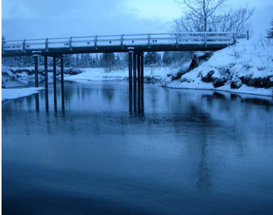
Appendix C2.—Looking upstream at the Lost River Road Bridge from discharge station 11702 on December 14, 2006 at a discharge of 49 cfs.
