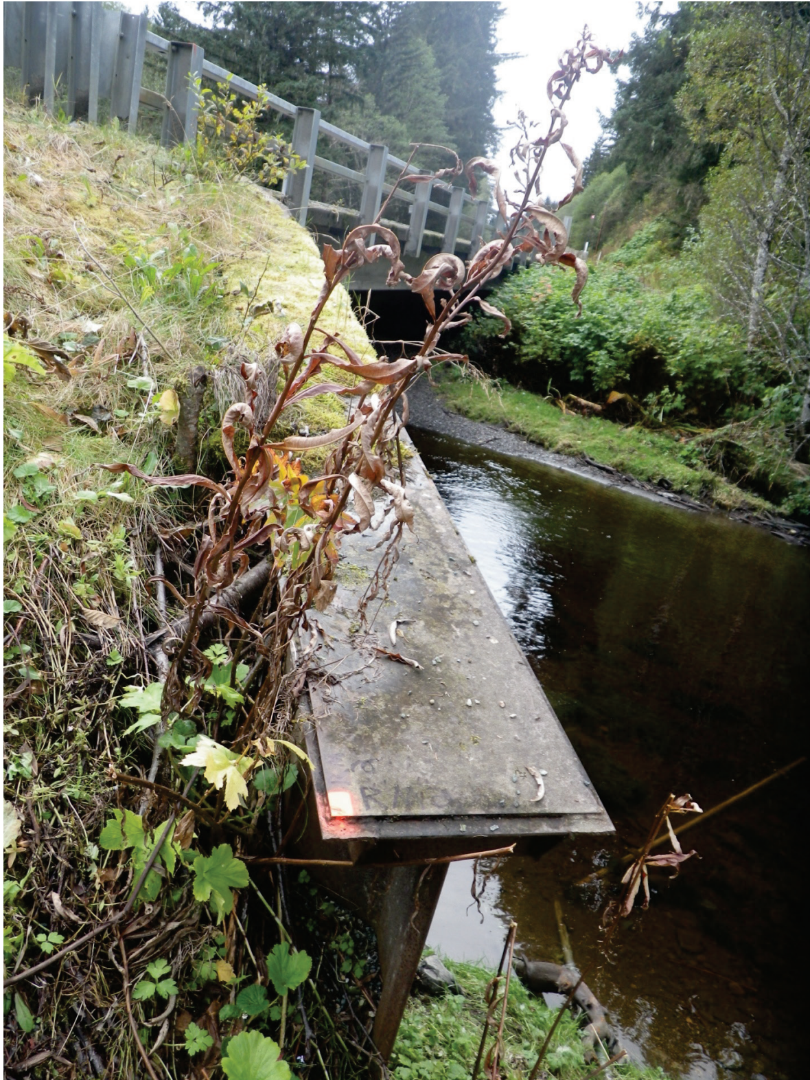
Figure 7.—Second water surface elevation marker (RM2) located at end of bridge abutment.
