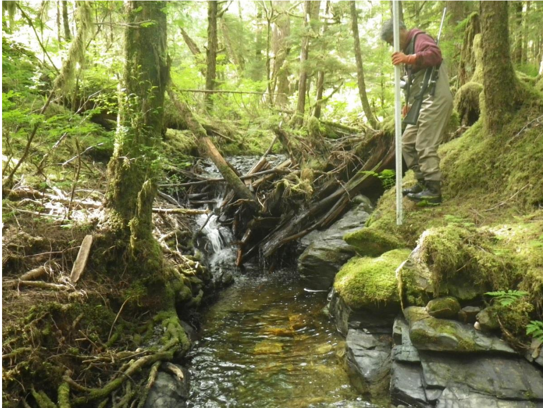
Photo 1: Trap Creek Tributary 1 barrier, that does not represent the upper extent of fish habitat.
