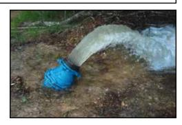
Poly Pigs run the pipeline, pushing debris, corrosion and mineral build up ahead of them until the lines are clean and operating at a much higher capacity.
