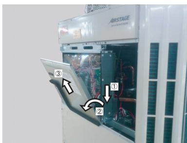
Remove the CONTROL BOX COVER
