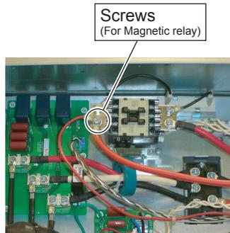
Remove the mounting screw and code.
