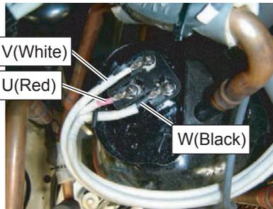
Remove the 3 mounting screws of Terminal.
