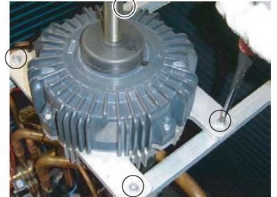
Remove the 4 mounting screws.
