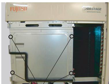
Remove the 4 mounting screws.
