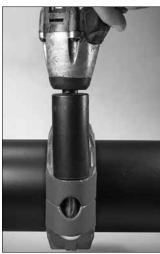
**6. TIGHTEN NUTS:** Tighten the nuts evenly by alternating sides until metal-to-metal contact occurs at the bolt pads. Make sure the housings' keys engage the grooves completely during tightening.
