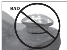
OVAL NECK OF BOLT NOT SEATED PROPERLY
