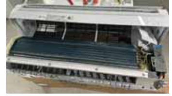
3. Remove the cover by removing these 10 screws.
