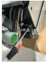
5. Remove leak sensor.
