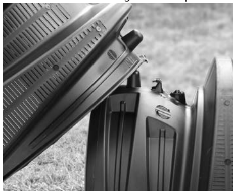
4. Connect the chambers.
