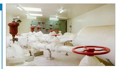
The Universal Air Valve is designed to permit the automatic escape of large quantities of air from a pipeline when the line is being filled, and to permit air to enter the pipeline when the line is being emptied. It also allows accumulating air to escape while the line is in operation and under pressure. This is accomplished with a compound lever system functioning in conjunction with a large and small orifice in one integral body casting.
