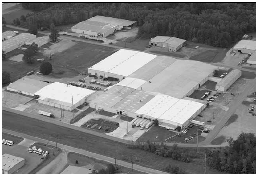
Ford Meter Box - Pipe Products Division Pell City, Alabama
