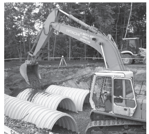
No equipment shall be operated on the bed at this stage of the installation. Excavators must be located off the bed. Dump trucks shall not dump stone directly on to the bed. Dozers or loaders are not allowed on the bed at this time.
