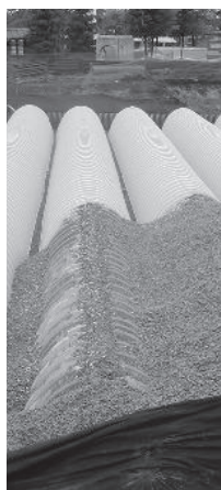
Initial embedment shall be spotted along the centerline of the chamber evenly anchoring the lower portion of the chamber. This is best accomplished with a stone conveyor or excavator reaching along the row.
