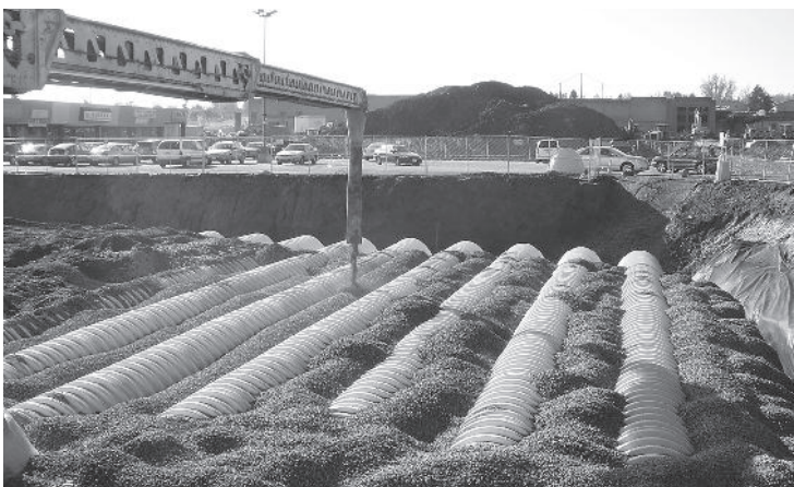
Initial embedment shall be spotted along the centerline of the chamber evenly anchoring the lower portion of the chamber. This is best accomplished with a stone conveyor or excavator reaching along the row.
