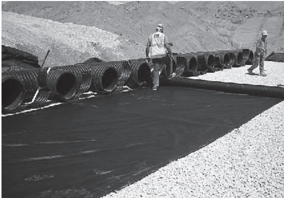
Install manifolds and lay out woven scour geotextile at inlet rows [min. 17.5 ft (5.33 m)] at each inlet end cap. Place a continuous piece (no seams) along entire length of Isolator® Row(s) in two layers.
