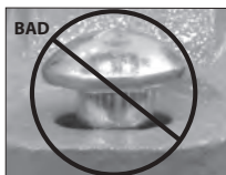
OVAL NECK OF BOLT NOT SEATED PROPERLY
