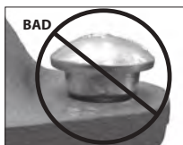
OVAL NECK OF BOLT NOT SEATED PROPERLY
