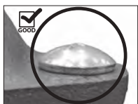
OVAL NECK OF BOLT SEATED PROPERLY
