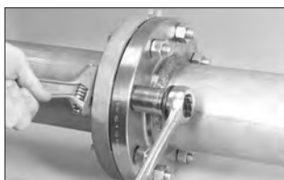
4-Bolt Tightening Pattern
