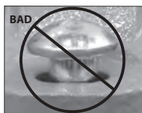
OVAL NECK OF BOLT NOT SEATED PROPERLY
