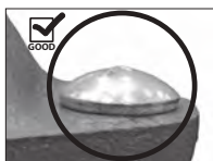
OVAL NECK OF BOLT SEATED PROPERLY
