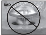
OVAL NECK OF BOLT NOT SEATED PROPERLY
