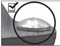
OVAL NECK OF BOLT SEATED PROPERLY
