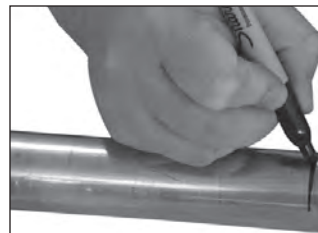
Figure 3 — Marking for Insertion Depth
