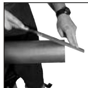
Figure 4: Deburr outside diameter using a half-round file
