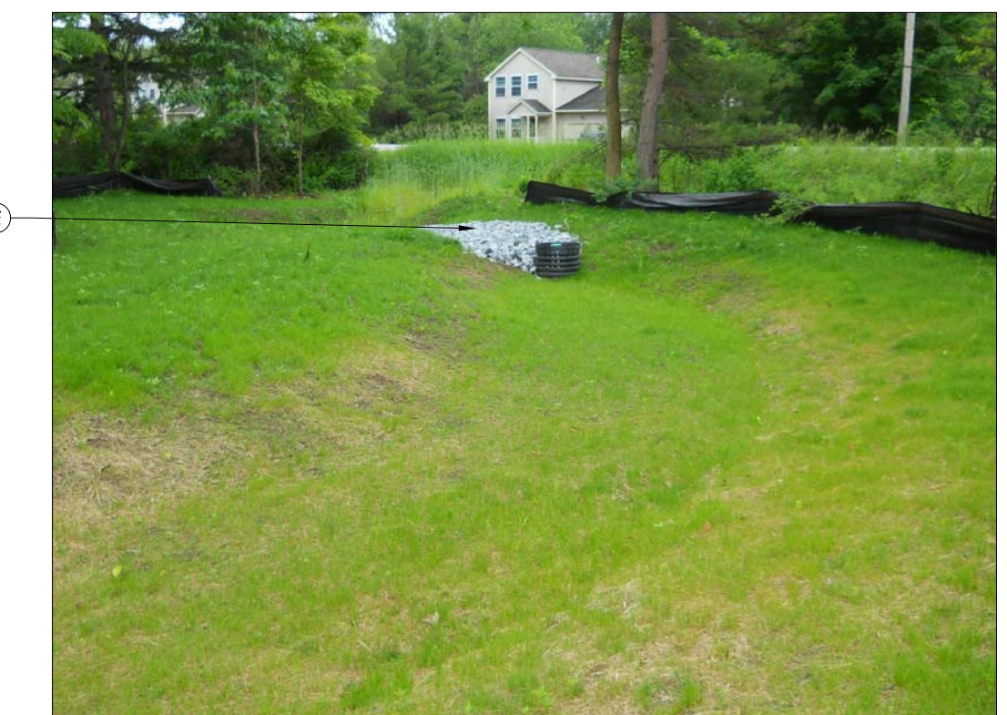
EXAMPLE OF AN 8' BOTTOM 2' DEEP SWALE
