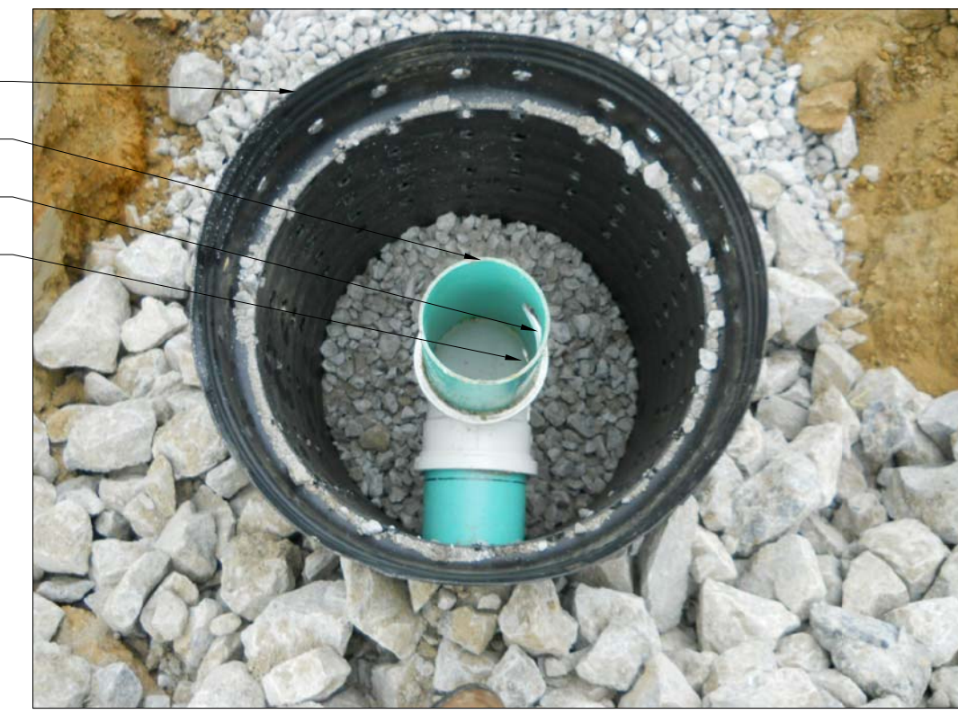
EXAMPLE OF A SWALE OUTFLOW DEVICE
