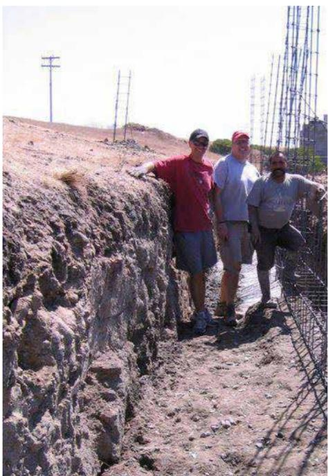
has been excavated so we are ready to begin the first floor. Our immediate need is to set pipes and electrical lines in place and pour the base slab.
