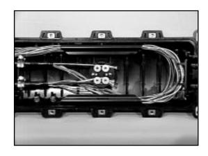
3.06 Trim the buffer tubes (without cutting the fibers) to the middle of the closure. Leave at least 75% of one coil buffer tubing intact.
