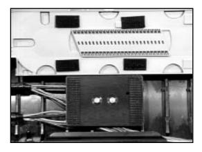
3.13 Center the tray over the adapter and press down to secure.
