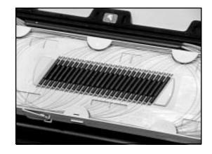
5.07 Install and close tray cover making sure that all fibers are properly stored under the tray tabs.
