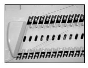
5.03 Place the splicing tool in close proximity to the splice tray. Prepare and splice the first pair of fibers.
