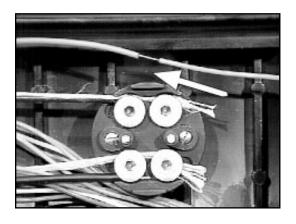
3.10 Slide the segment of tubing over the buffer tube about 1" (25 mm) and secure with two wraps of vinyl tape.
