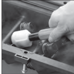
Installation of Hardened Connectors
