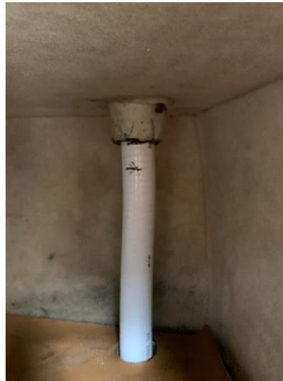
We reamed out the hole in the fiberglass with rotary rasp so the tubing would slip through. Flared the top of the hole a bit to receive epoxy resin that would seal around the tubing and ooze down between the tube and the fiberglass. Putty was placed around the internal end of the joint to prevent the epoxy from running out. The resin was delivered to the flared opening at the top of the tube/fiberglass joint by pouring it down a PVC pipe/straw.
