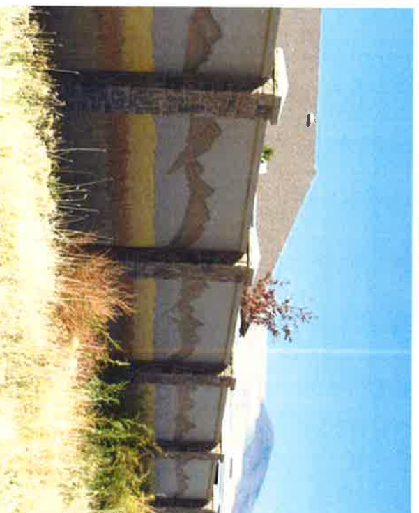
6' Standard Herriman Wall with 2' Berm (Installed on top of Berm)
