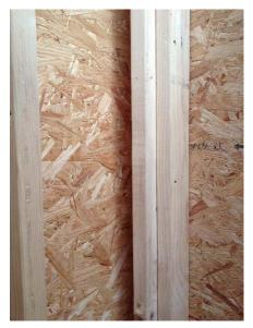
The corner posts are framed in a way that allows the wall insulation to fit behind the corner posts, so as not to lose air at the corners. This is also above and beyond the local building code requirements.
