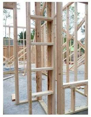
T's at 90 degrees wall intersections: this is a photo taken from outside the home looking in – These intersections are framed in a way that (like the corner posts) do not allow for an air pocket to exist, therefore there cannot be an air pocket without insulation. The intersection is framed in a way that allows wall insulation to fit behind this "T post," which results in less air loss, which results in a lower power bill, and a stronger build.
