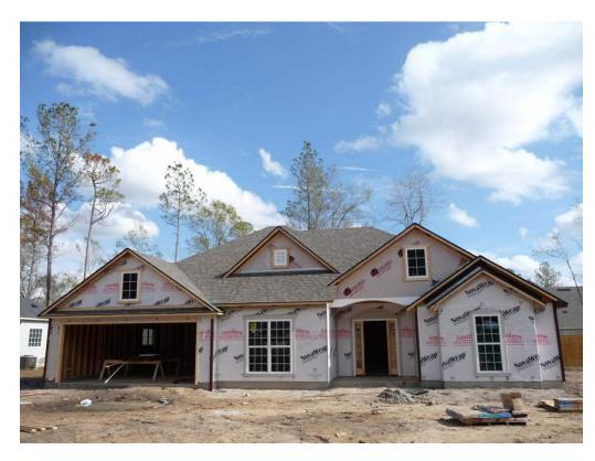
The house is wrapped with a product that moisture allows to through and pass dissipate, but not air, similar to the higher exercise end and sporting gear available today, designed to keep your body dry as you build up heat and perspire.
