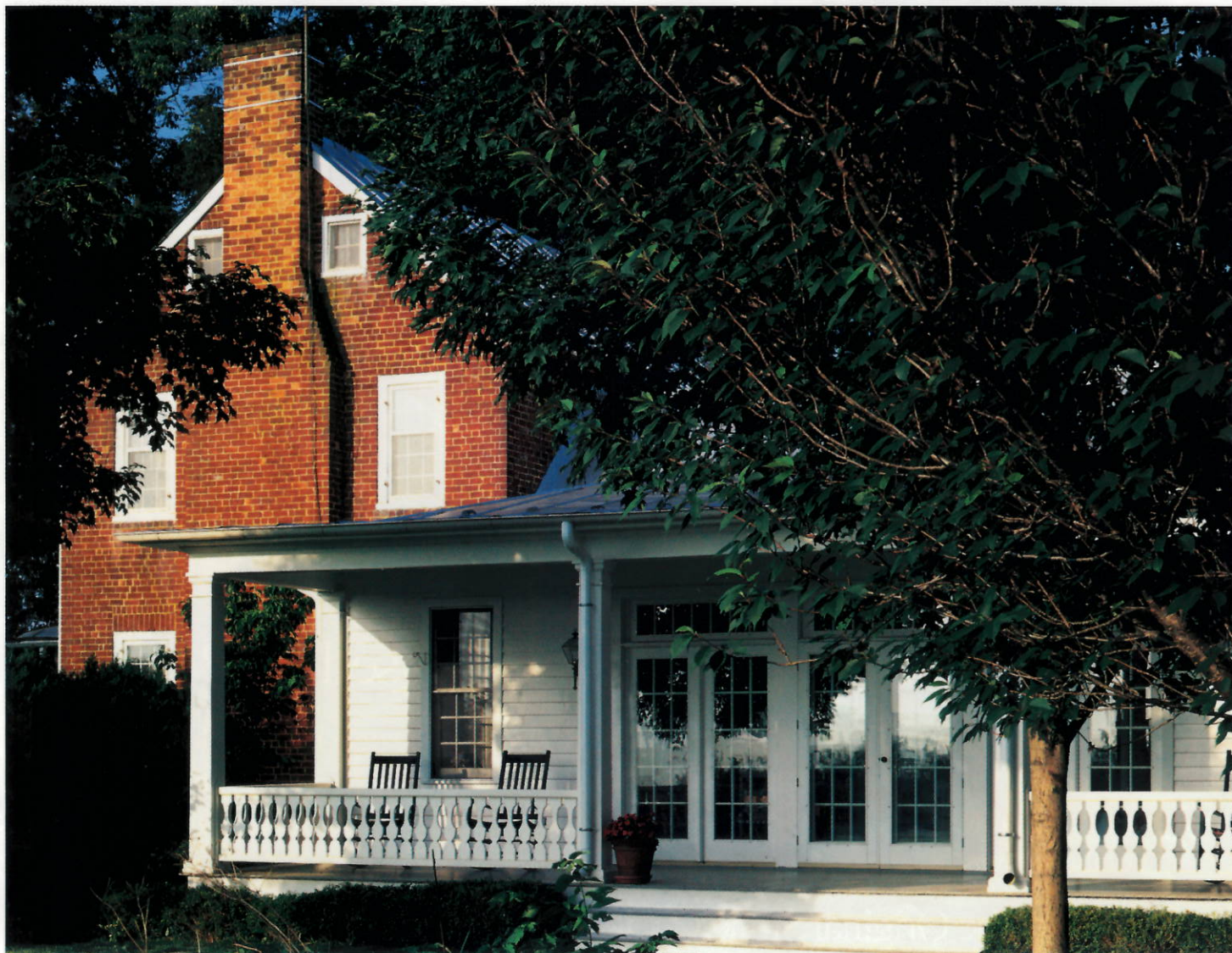
Frazier Associates blends old and new seamlessly in this porch addition on a nineteenth-century farmhouse in Virginia's Shenandoah Valley.
