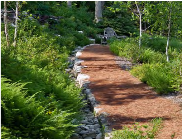
Infiltration trench parallelling a pathway.
