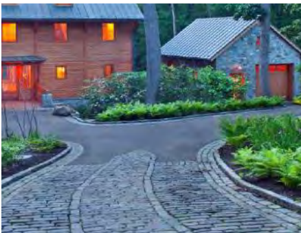
Banding asphalt driveway with stone.
