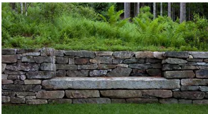
Simple bench constructed of indigenous stone.
