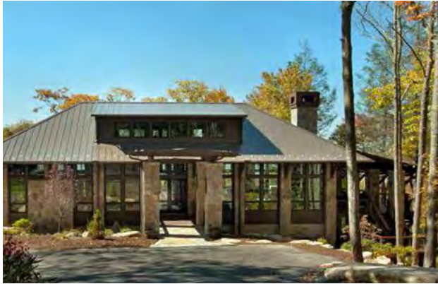
Standing seam metal roof with low sheen.
