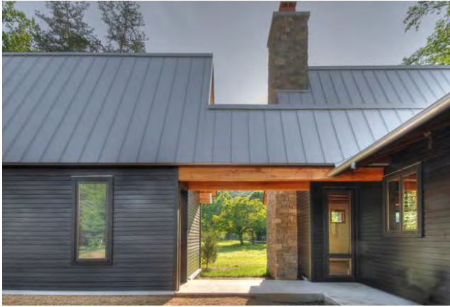
Wood siding oriented horizontally.
