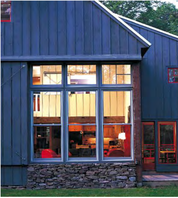
Fiber cement board siding with vertical battens.
