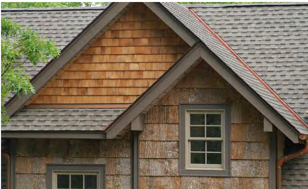
Natural bark siding and natural shingle siding.
