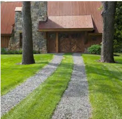
Tire track driveway reduce impervious service.
