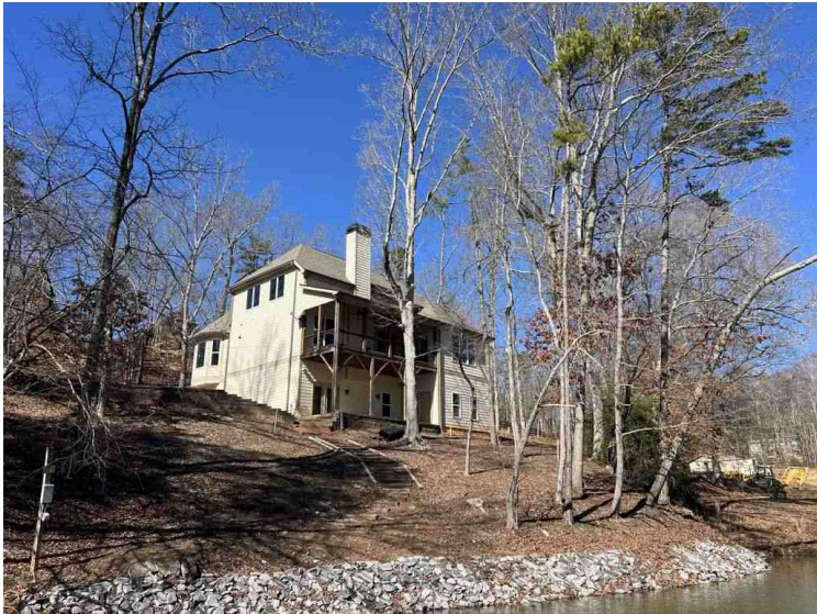
View of subject from dock
