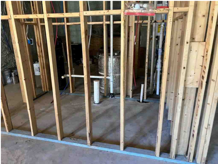
Unfinished basement - stubbed for bath
