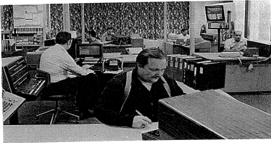
Figure 15-3. A typical Switching Control Center. One of New York Telephone's Switching Control Centers is the hub of local switching office surveillance, testing, and maintenance for over a dozen central offices. Switching equipment technicians are assisted in their work by computer-based operations systems.
