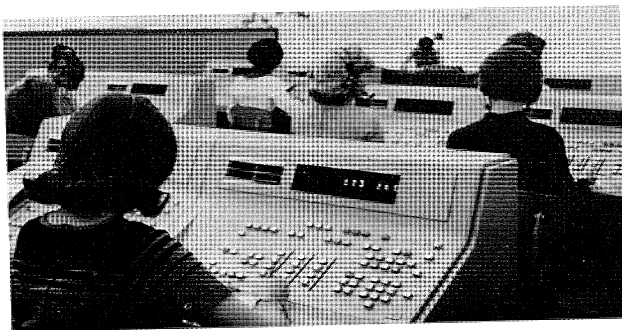
Figure 10-16. A typical TSPS operating room.
