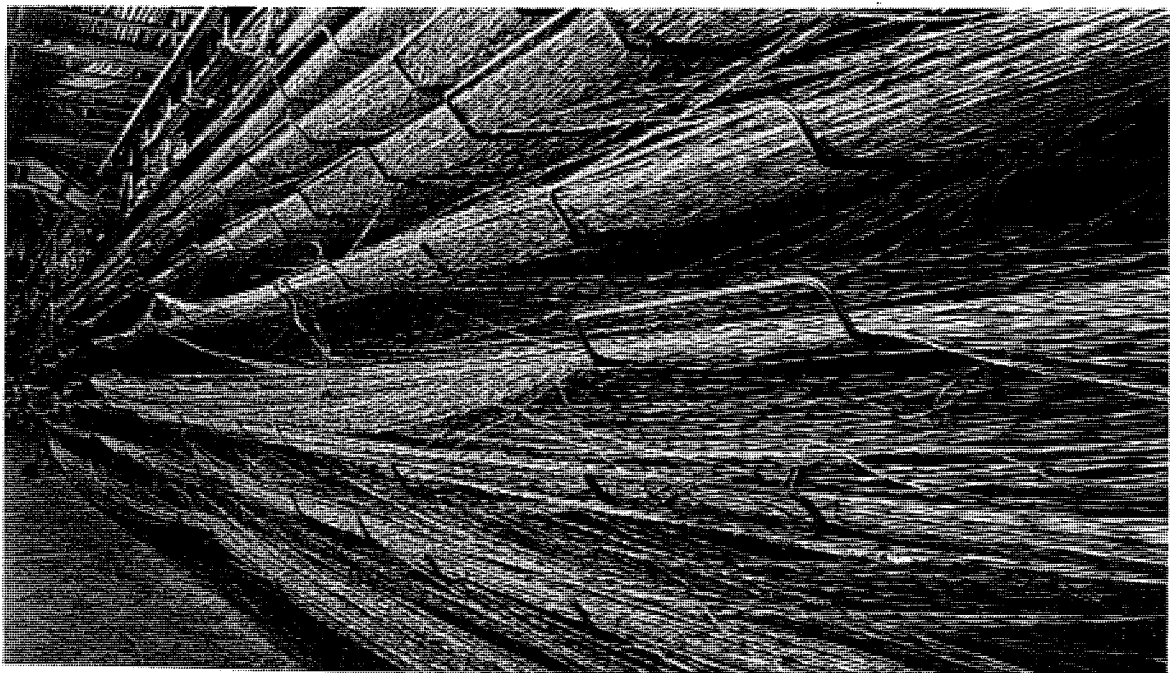
Figure 12-10. An overloaded main distributing frame in a central office.
