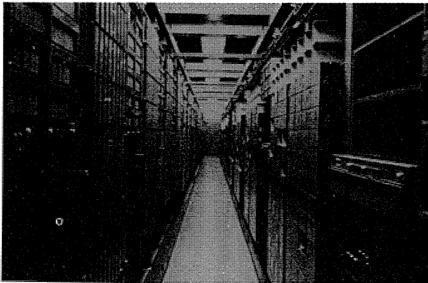
Figure 12-15. Equipment frames in telephone equipment buildings. A , transmission equipment; B , crossbar switching equipment mounted on 11-½ foot high framework lineups; C , ESS switching equipment mounted on 7-foot high framework lineups.
