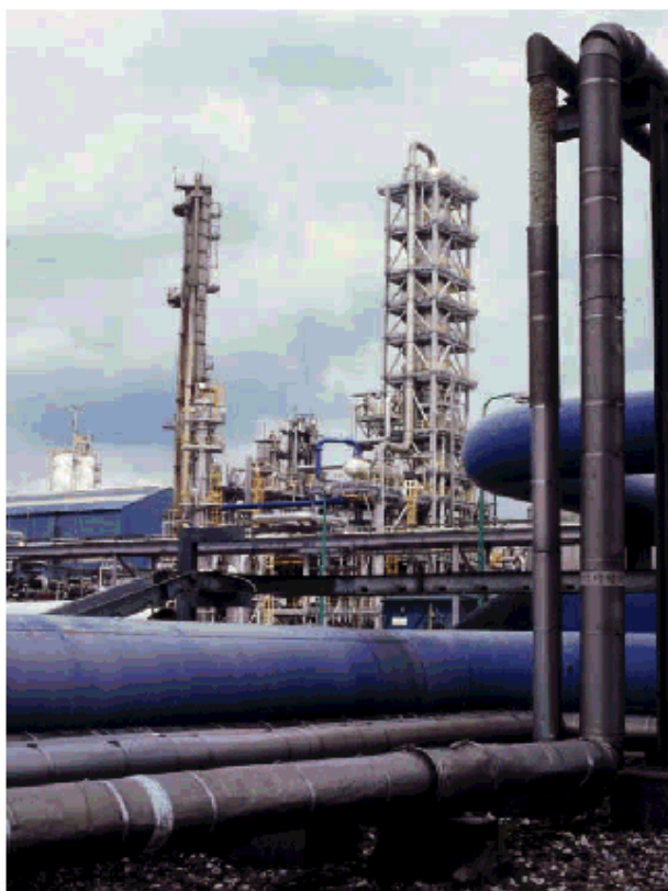
Fig. 1 The Cativa™ acetic acid plant which is now operating at Hull. The plant uses a promoted iridium catalyst package for the carbonylation of methanol. The new combined light ends and drying column can be seen
