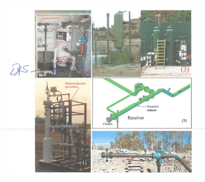
194. This group of photographs show that there is absolutely nothing the least bit unusual or unique about changing the diameter of a pressure vessel, and that the method of accomplishing the diameter change can be done with fittings (either eccentric or concentric) or by modifying a pressure vessel fabricated head. Modifications to the pressure-head can be done in any orientation required by the process. There are common welding templates for creating a concentric connection
