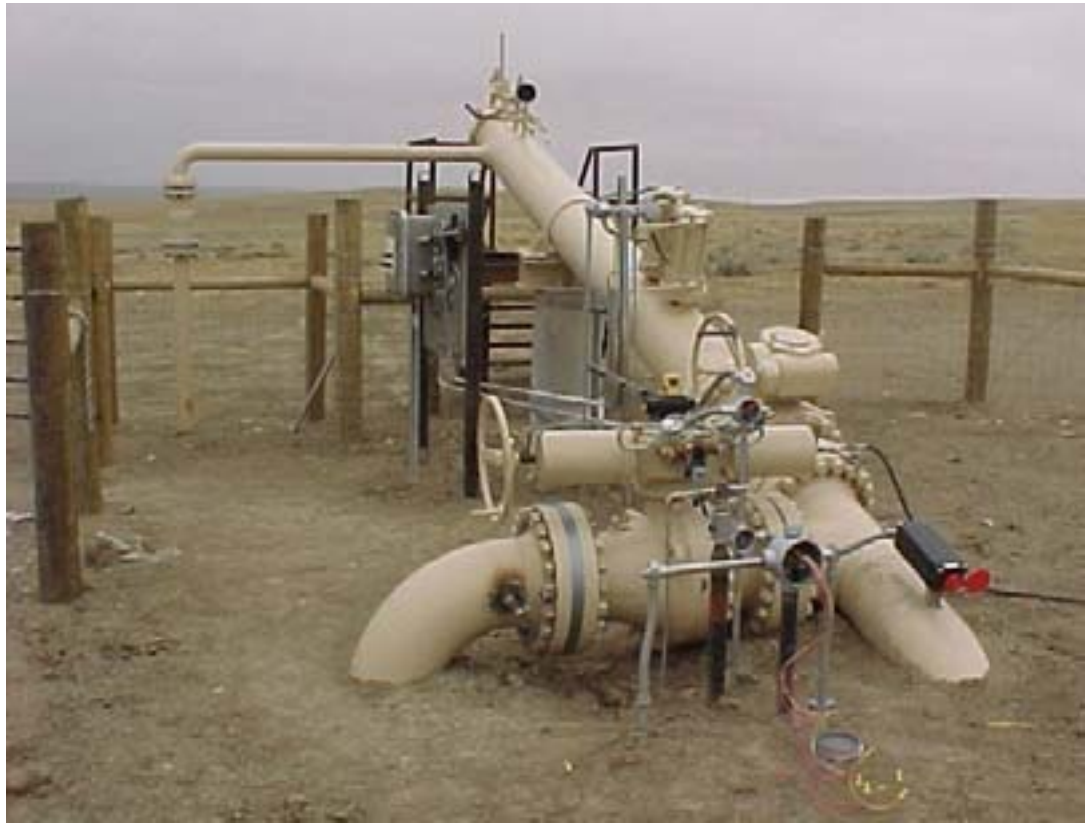
Figure 3 – Automatic Ball Launcher
