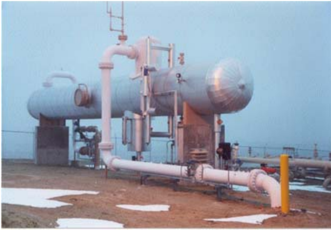
Figure 18 – Complete Slug Catcher Installation
