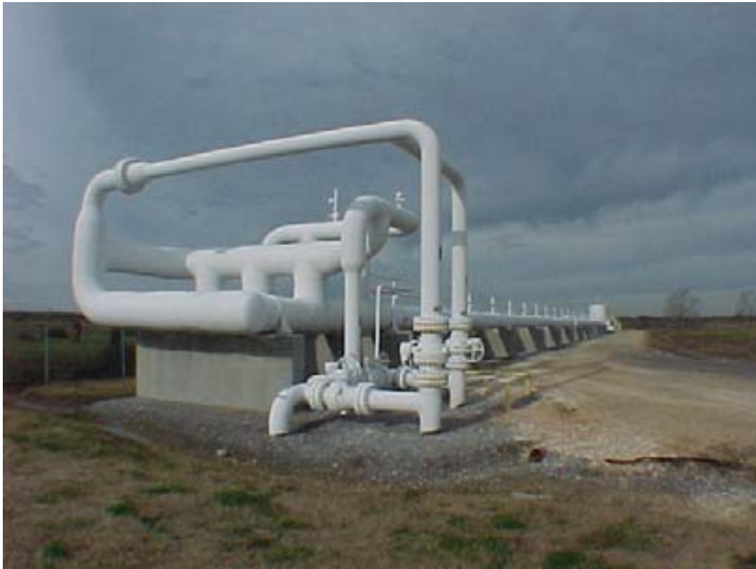
Figure 14 – Slug Catcher – Inlet End View
