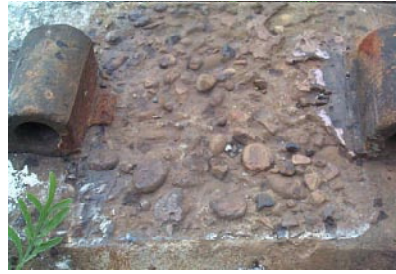
Figure 2. Rail seat abrasion due to water intrusion (Peters 2003)
