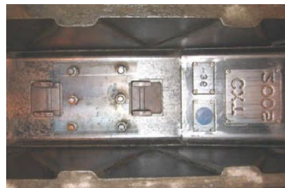
Figure 6. Steel plate to be cast-in prior to casting (Peters 2003)
