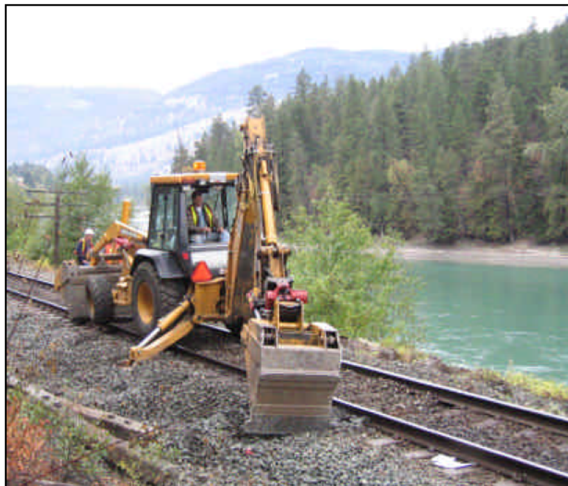
Figure 11 – Hi Rail Backhoe Replacing Every 6 th Tie in Front of Main Gang
