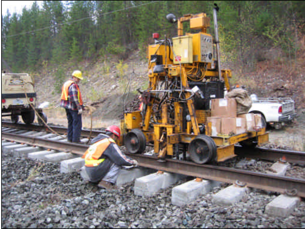
Figure 14 – Pad Installation
