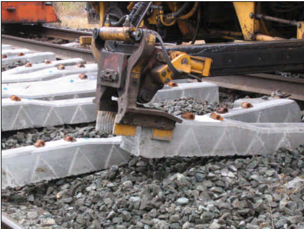
Figure 13 – TR-10 Tie Insertion
