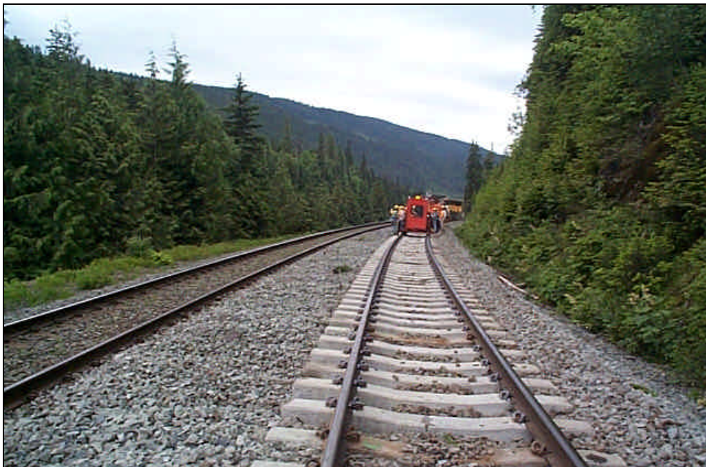
Figure 17 – Track Clipped and Ready for Ballast and Final Tamping
