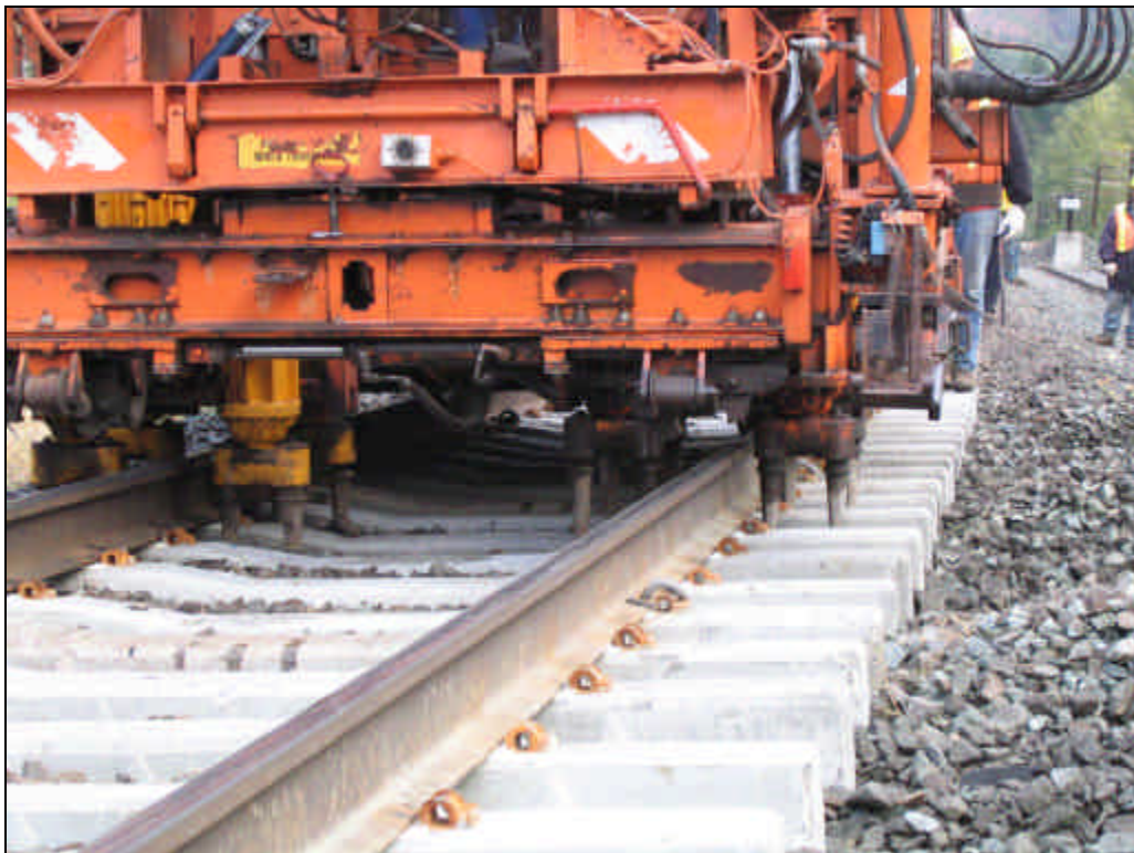
Figure 15 – First Pass Tamp to Nip Ties
