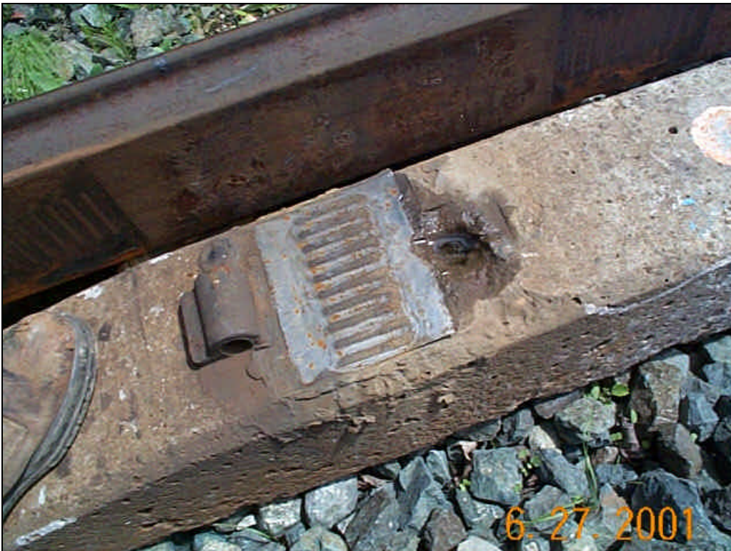
Figure 4 – Tie with Broken Ductile Iron Shoulder
