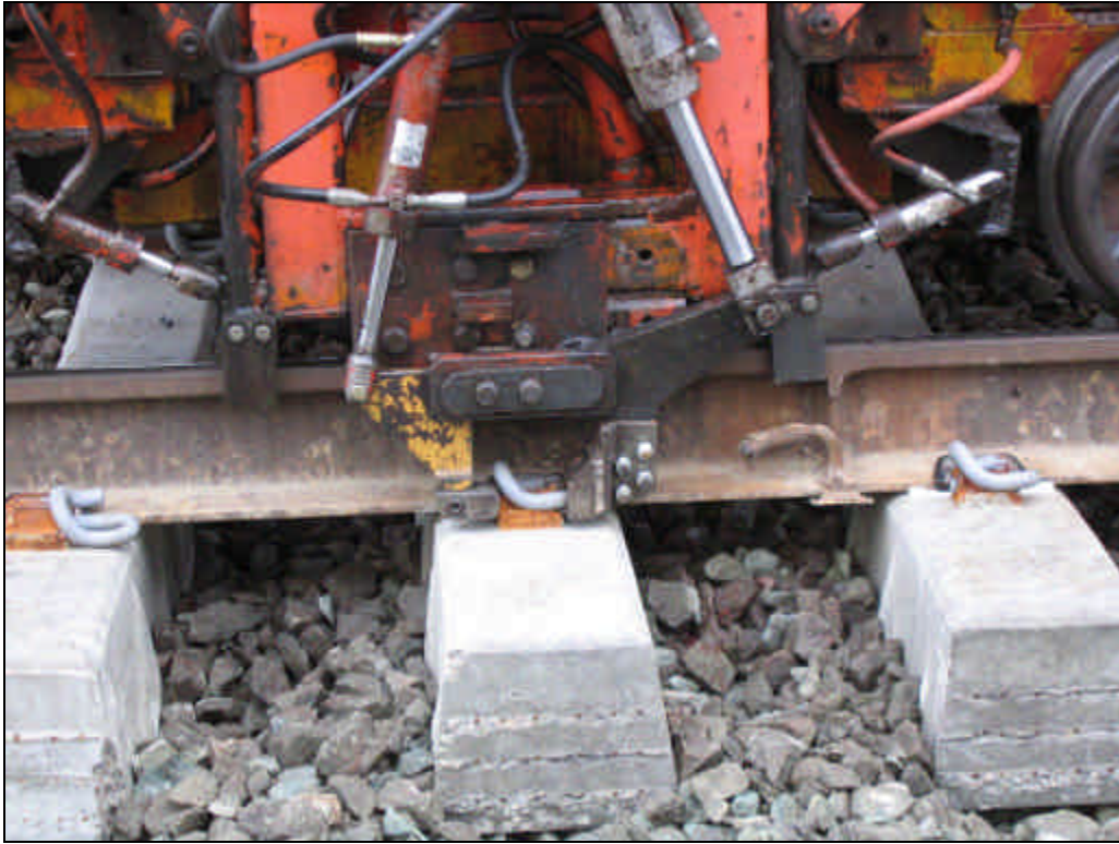
Figure 16 – Clip Installation
