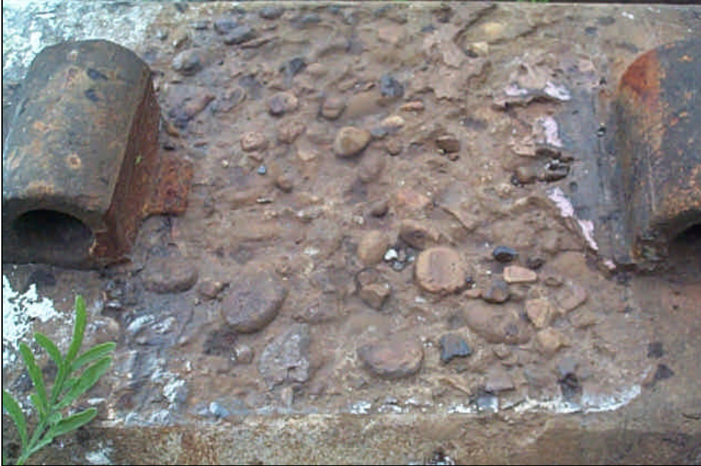
Figure 3 – Railseat Abrasion
