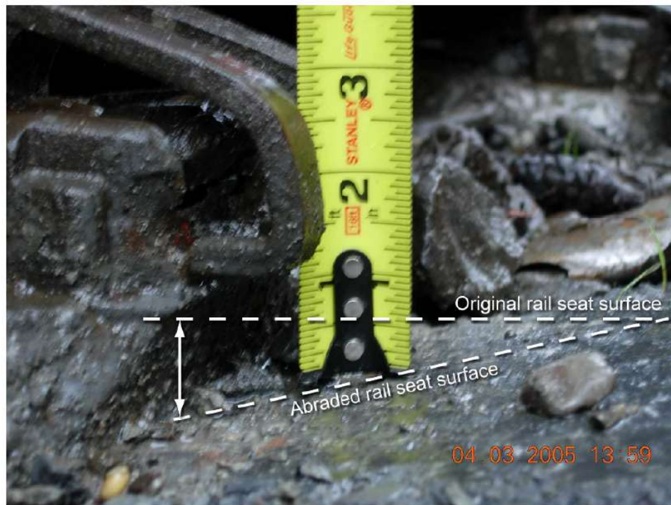
Figure 5. Concrete crosstie abrasion of about 1 inch at derailment site.
