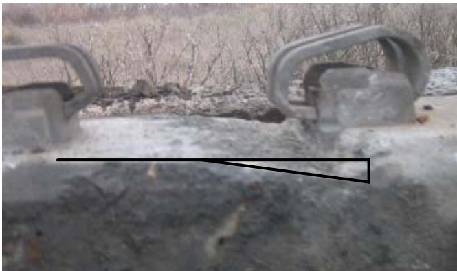
Figure 1. Triangular abrasion pattern in a concrete tie with black lines outlining a triangular pressure distribution assumed for this analysis.
