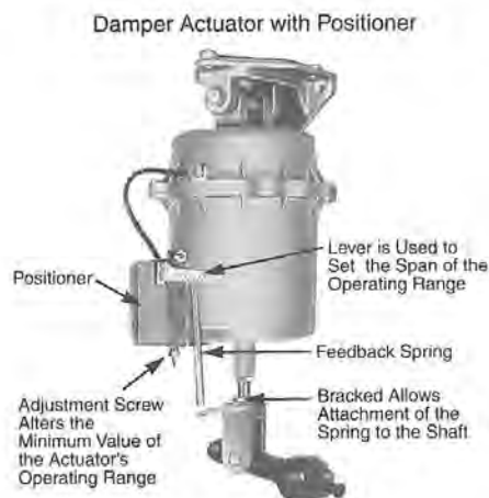
Figure 10.3 Positioning Relay and Damper Actuator
