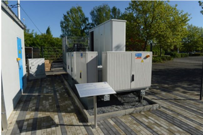
Fig. 16. GE 1MW SiC inverter installed in Berlin.
